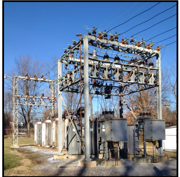
The Fuller Street substation is currently a 2400 volt station with equipment dating back to the 1940s & 1950s.
