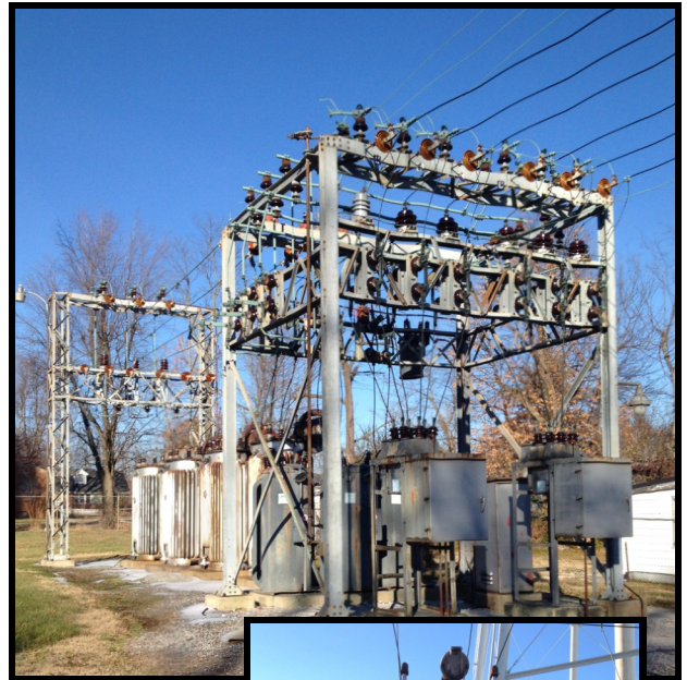
The Fuller Street substation was a 2400 volt station with equipment dating back to the 1940s & 1950s.
