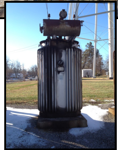
The Fuller Street substation was a 2400 volt station with equipment dating back to the 1940s & 1950s.
